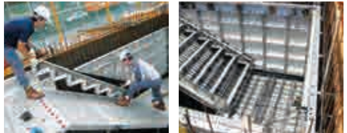
+4 Installation of staircase panels
