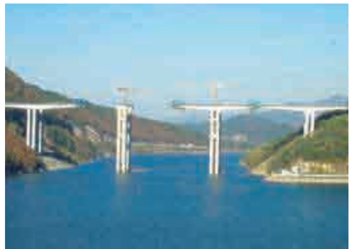
+ Shindanyang Large Bridge - Korea
