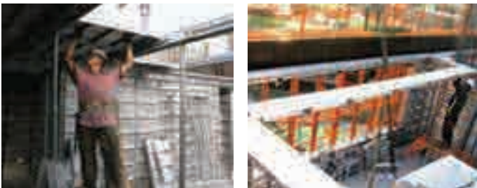
+5 Installation of slab panels
