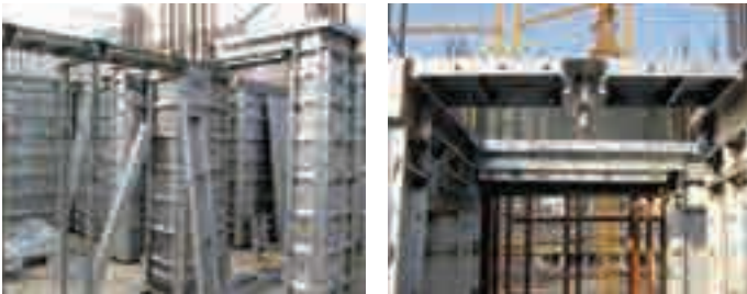
+3 Installation of beam and SC panels
