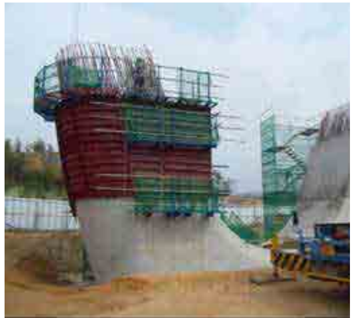
+ 4th Geumgang Bridge - Korea
