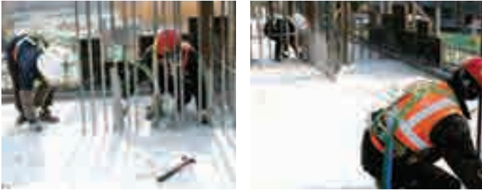
+1 Structural line and level check
