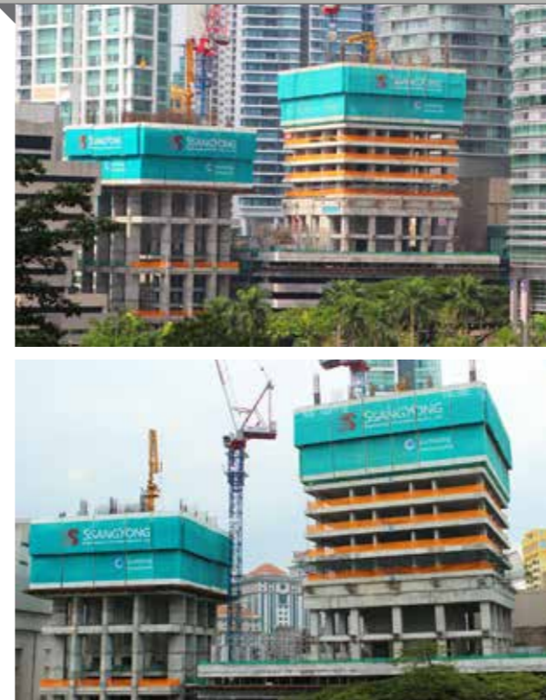
DNP Tower, Kuala Lumpur - Malaysia
