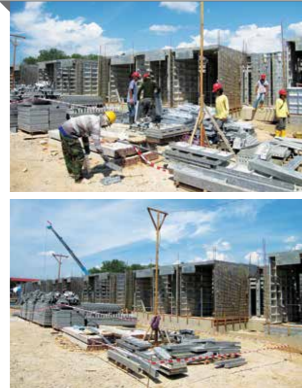
Universe Prime Condominium, Sabah - Malaysia
