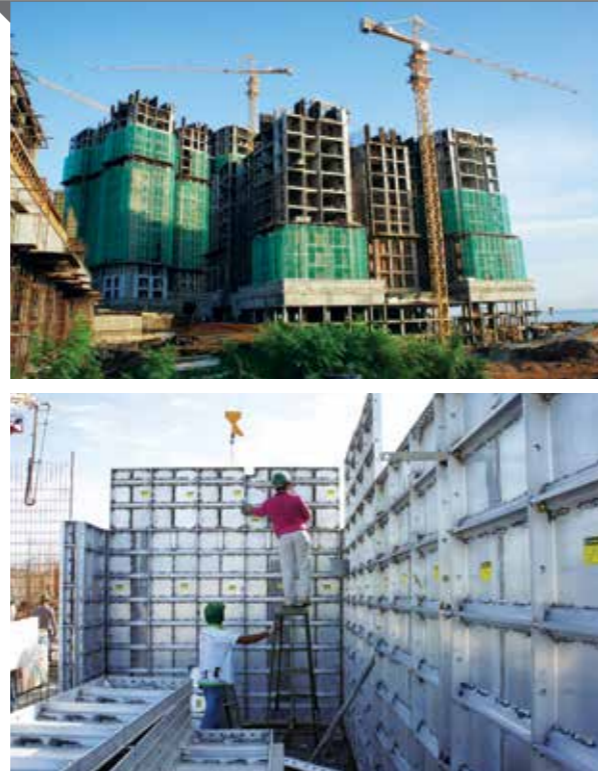
STP Condominium, Kuala Lumpur - Malaysia
