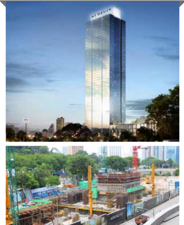
ONE IFC Tower, Kuala Lumpur - Malaysia
